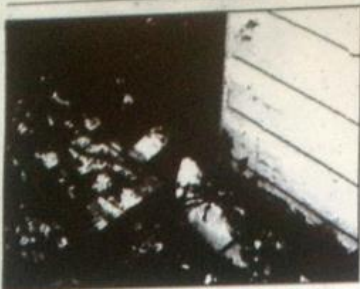
RUBBLE PIT: A fairly typical rubble pit in Wagga. Stormwater is directed into the ground through a downpipe at the back of homes.
